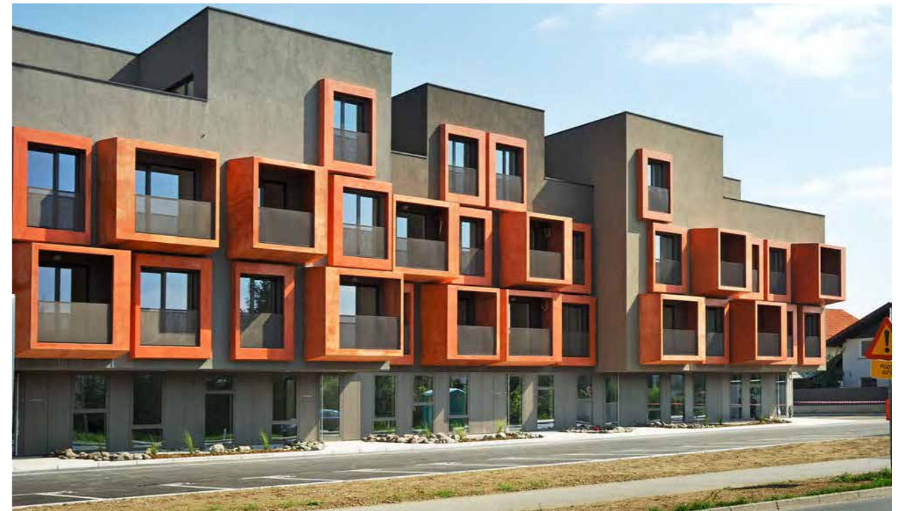
Jamaica Townhouse Apartment Project
